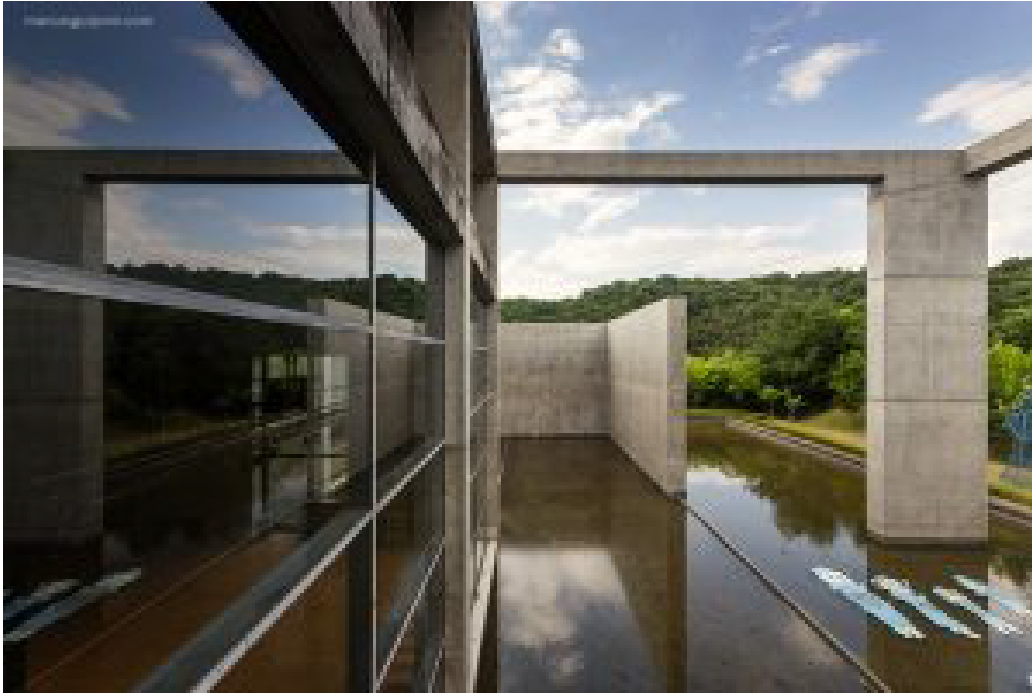
View of the water terraces outside the multipurpose hall and library (from Google Maps)
