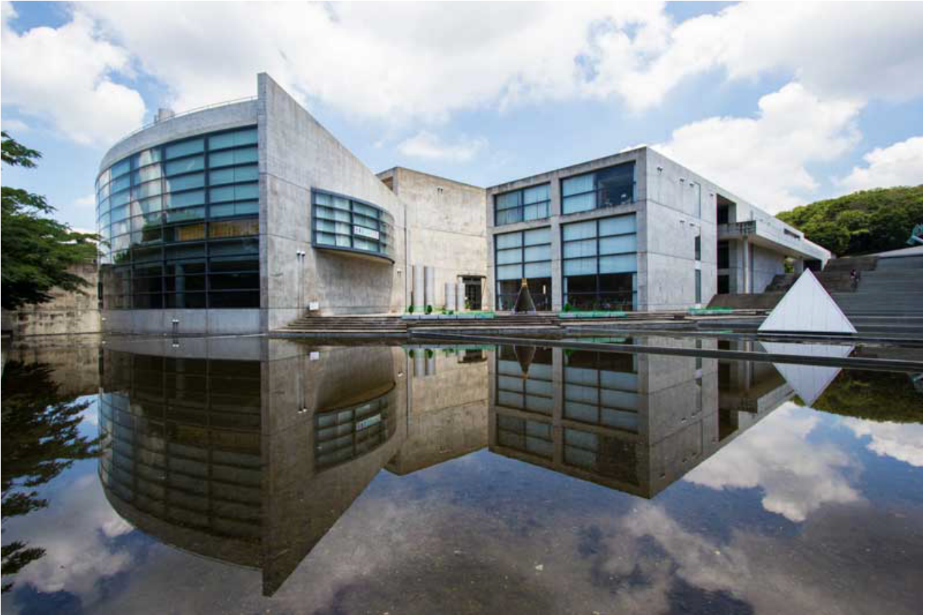
Perspective view of the building's south west corner (from Google Maps)
