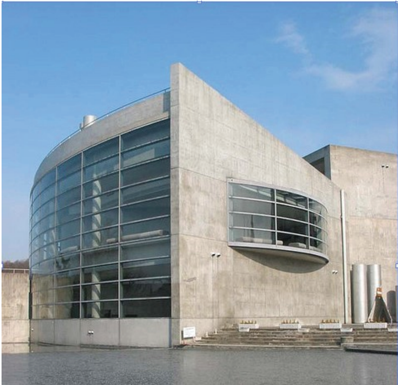
View of the fan-shaped wing and its curved glass elevation (from Google Maps)
